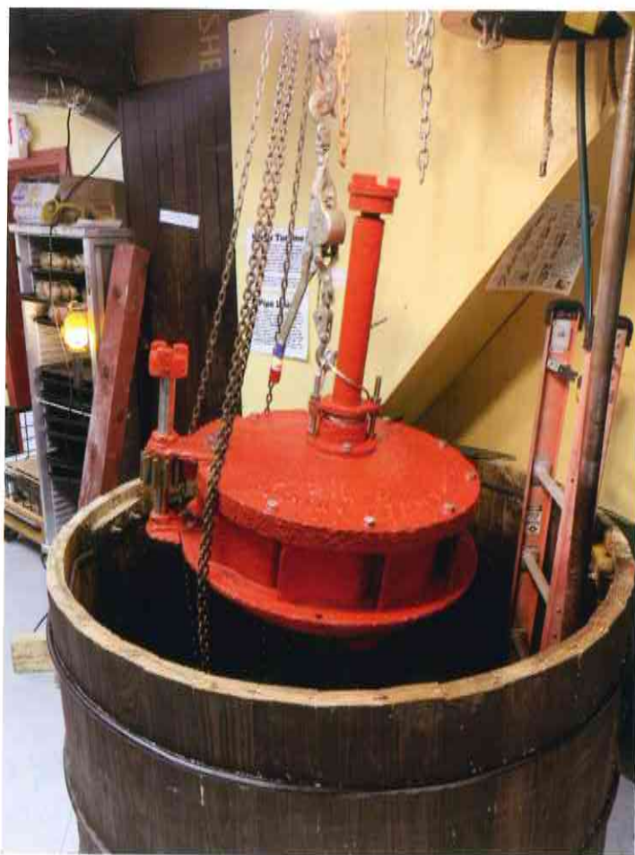
Turbine being lowered into the shaft.
