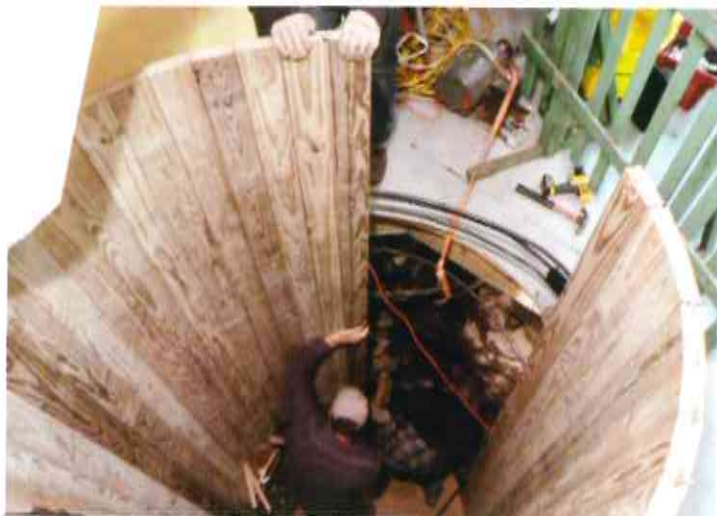
Crew working on shaft for tank replacement
